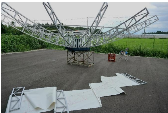
Early 2021, 6-m truss section was started.
