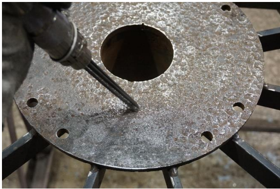
Rust was removed using air-powered chisel.
