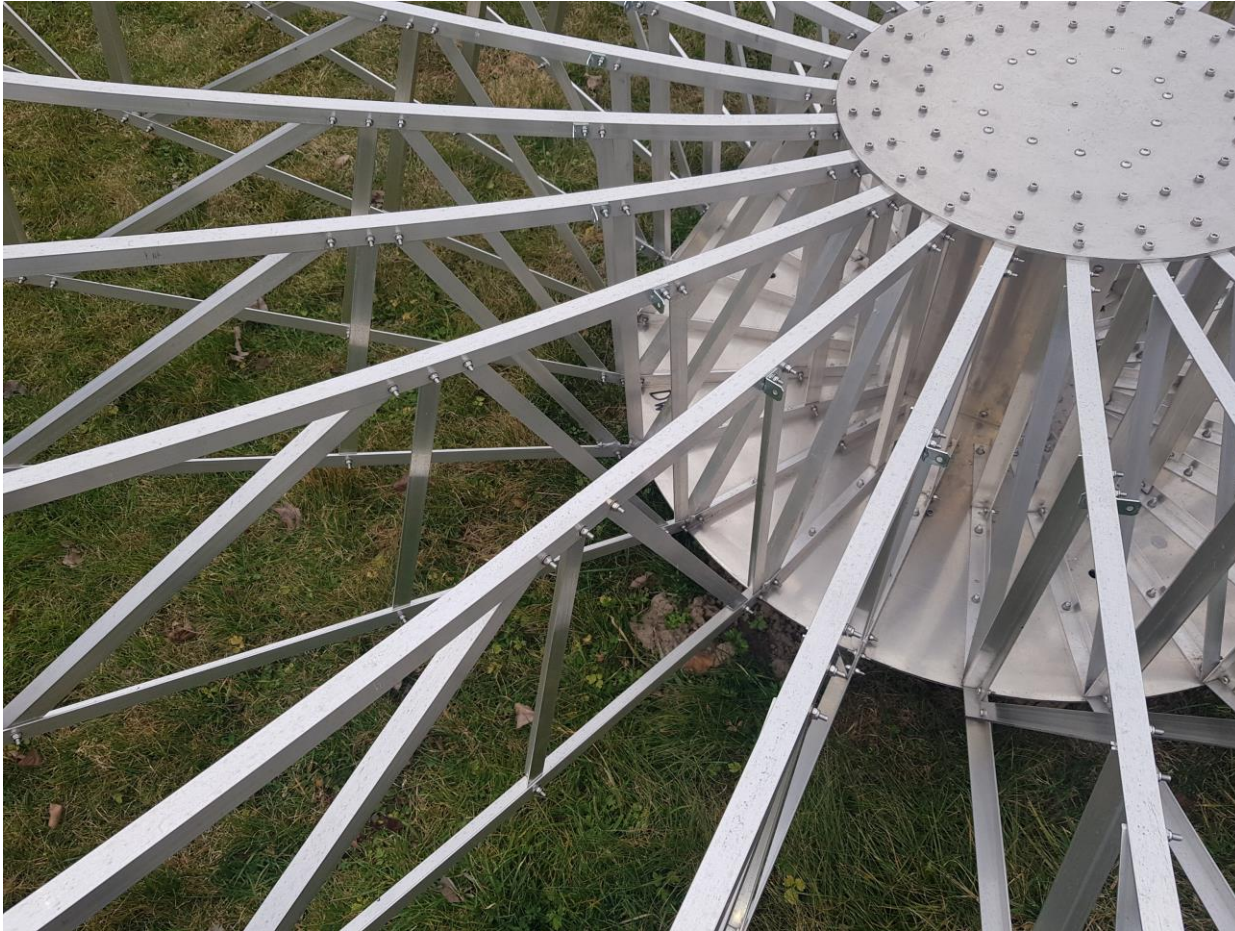
All of ribs are screwed with stainless steel screws.
