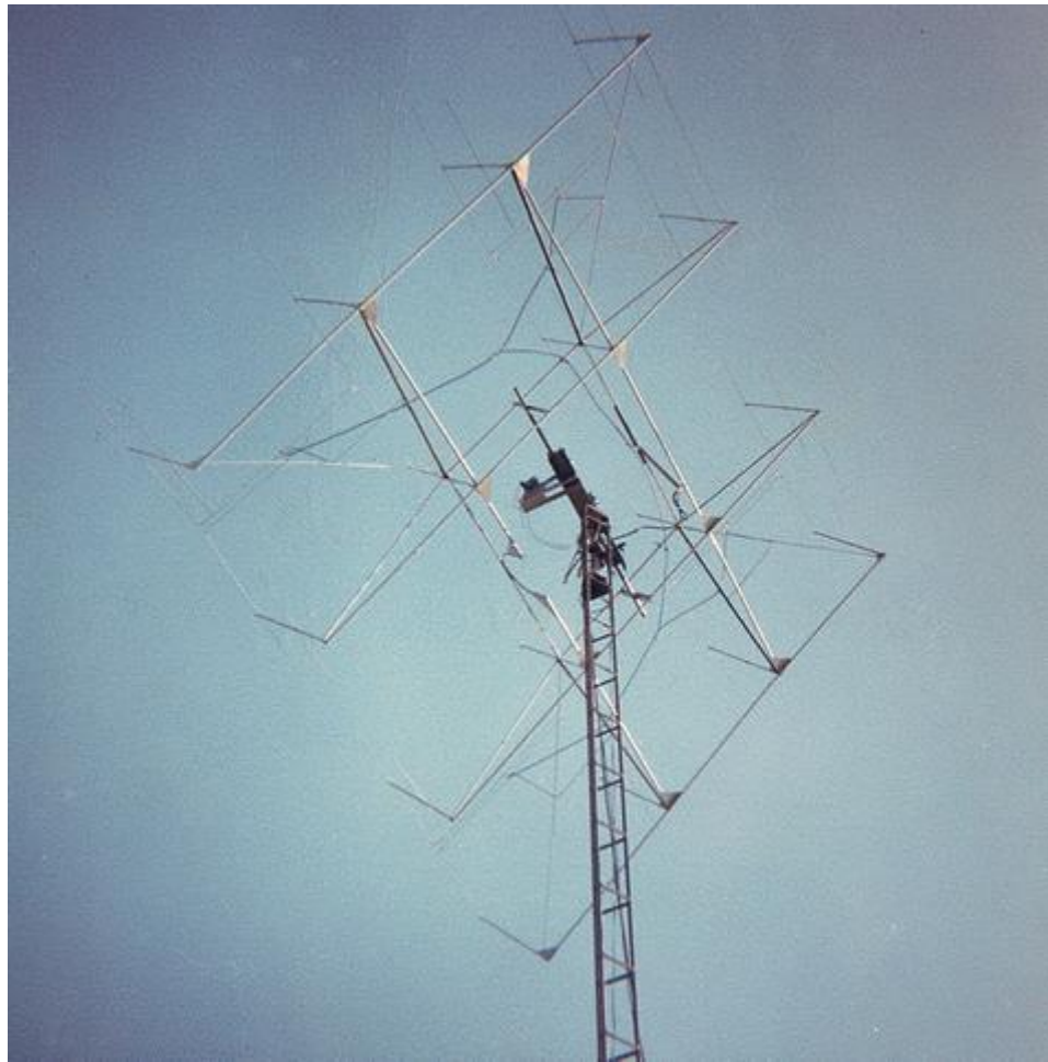
This is the 32-element expanded-extended collinear array at W6DNG, Long Beach, California. (W6DNG photo, tnx for F8DO)
