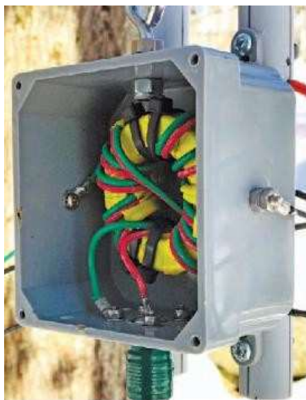
Photo 1.1.5.3. Junction box with symmetriser and two PVC struts
