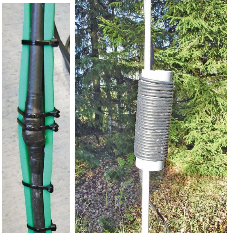
Photo 1.2.9.4. As reinforcement of the connections there are plastic cups to which the ends of the cables are tied by ties.
