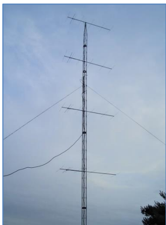
4 x 7 element fixed direction HB9 and I
