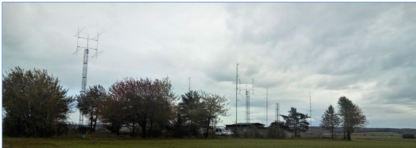
An overview of the antenna farm at JN38AT (Rosières-en-Haye) in about 310 m a.s.l.
