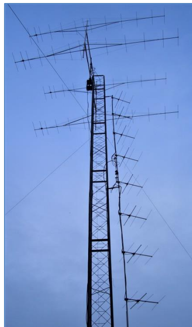
Two systems at only one tower On top: The 4 x 12 element rotatable Below: The 8 x 4 fixed direction North DL and Benelux
