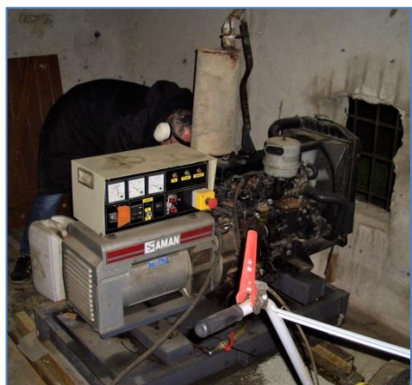
Like at the F6KFH site, and unusual for France: Electricity generated NOT by nuclear power
