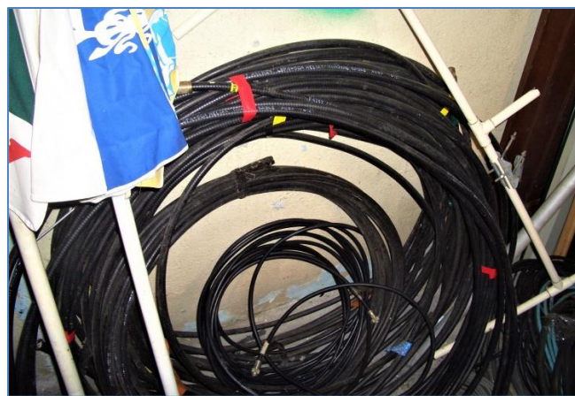
After all the antenna building it seems that still some hardwire coaxial cable is left as spare
